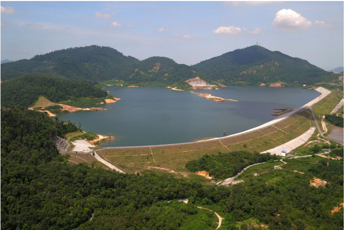
Mengkuang Dam is the largest dam in Penang and serves as a strategic drought reserve.
