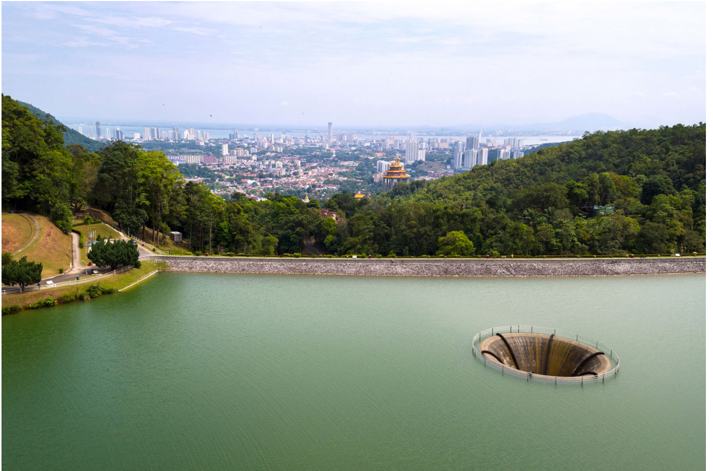
Air Itam Dam, Penang. © PBAPP 2019
