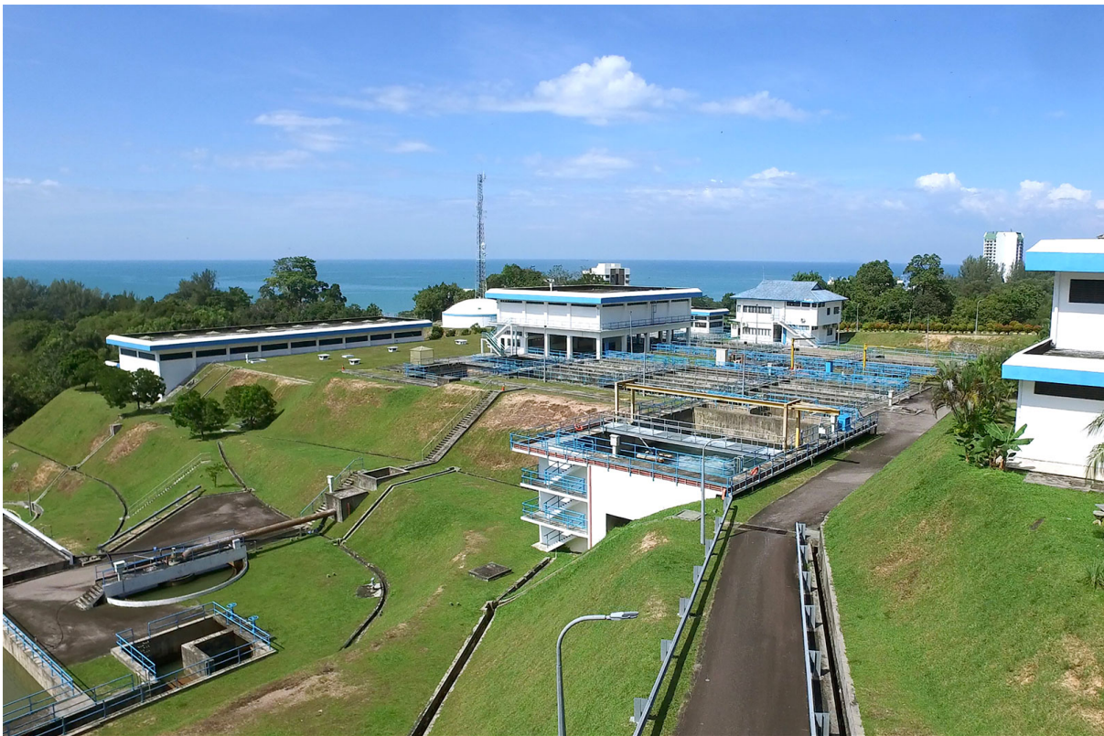
Batu Ferringhi Water Treatment Plant, Penang Island, Penang.
