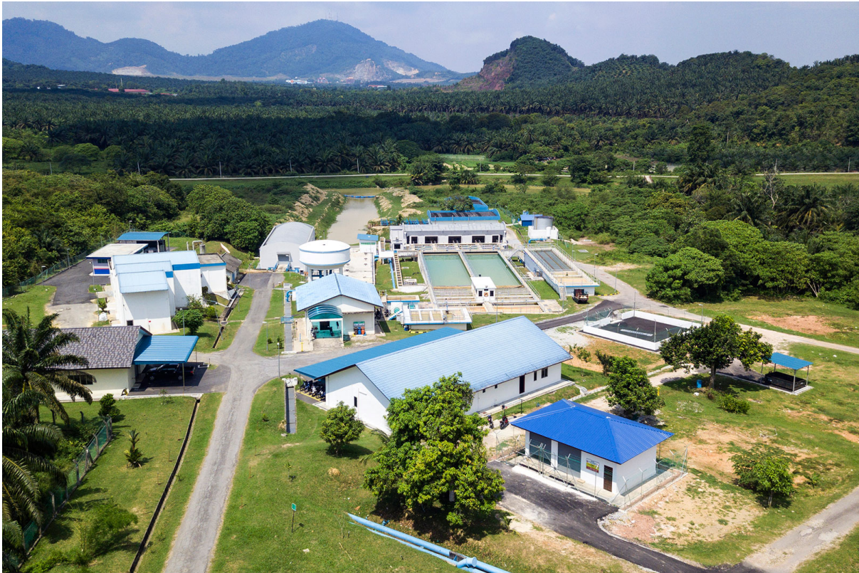
Bukit Toh Allang Water Treatment Plant, Ara Kuda, Seberang Prai Utara, Penang.
