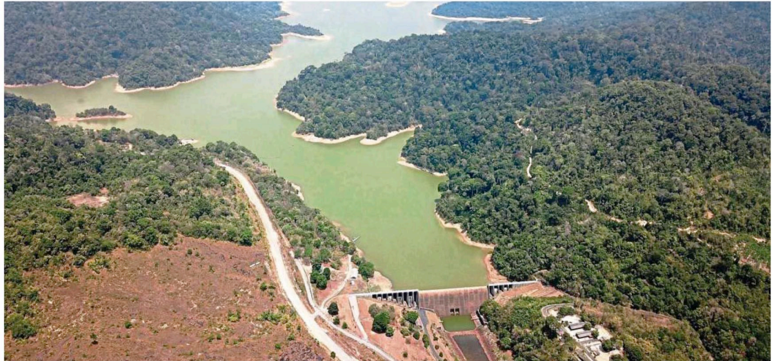
An aerial view of Ulu Muda Lake in Kedah with the dam (at bottom right of picture). – Filepic
