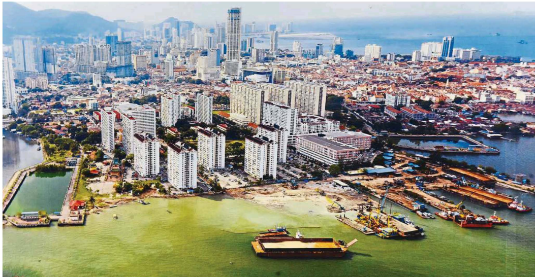
A view of the Macallum seafont where excavation and land reclamation works for the third Penang submarine pipeline have been put on hold voluntarily by the contractor.
