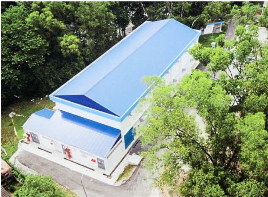
A general view of the RM11.9mil station in Bukit Dumbar.
