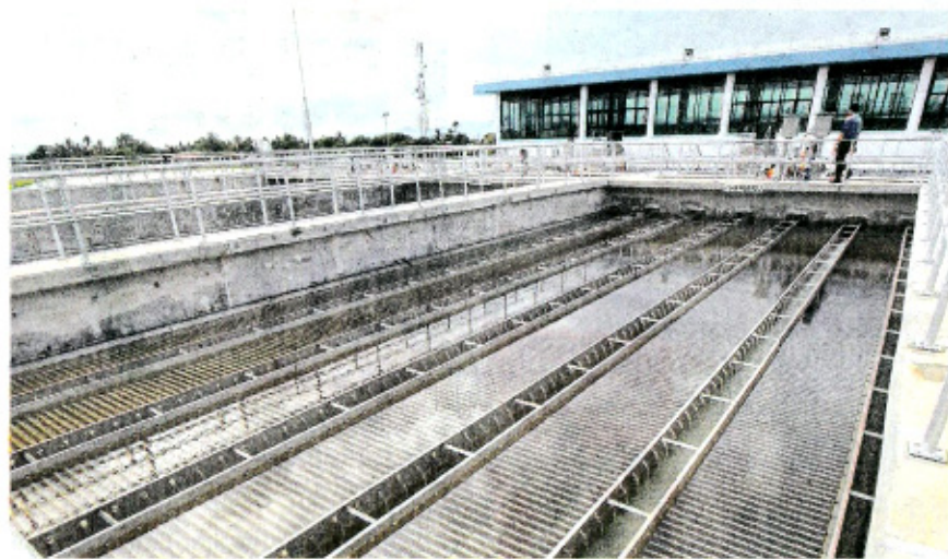
The residue produced by the Sungai Dua Water Treatment Plant can now be recycled into a material for making clay bricks.
