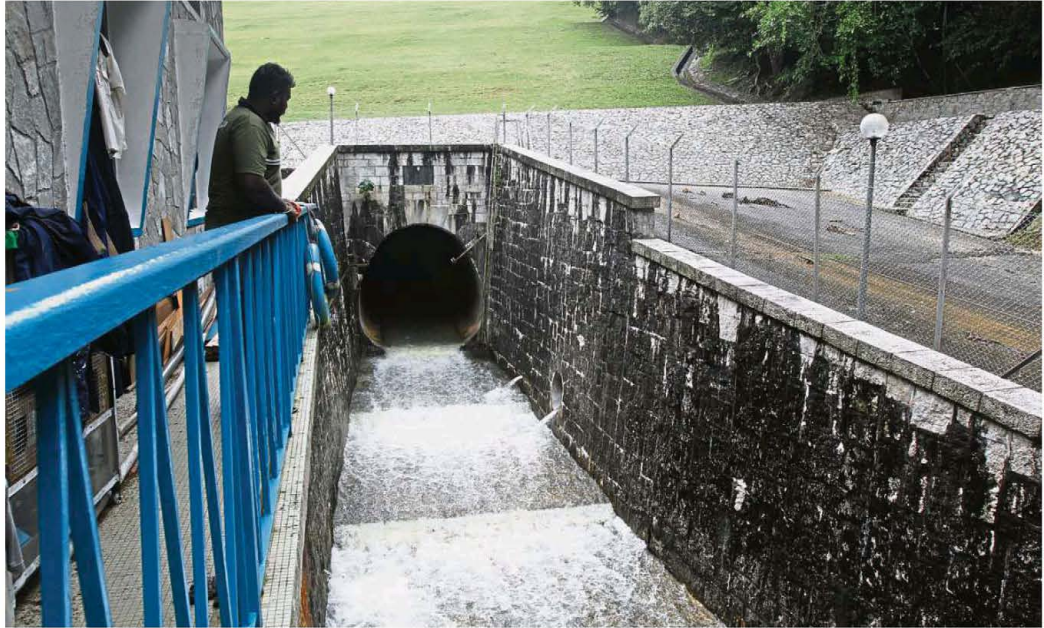
Water being released at the spillway at Air Itam Dam.
